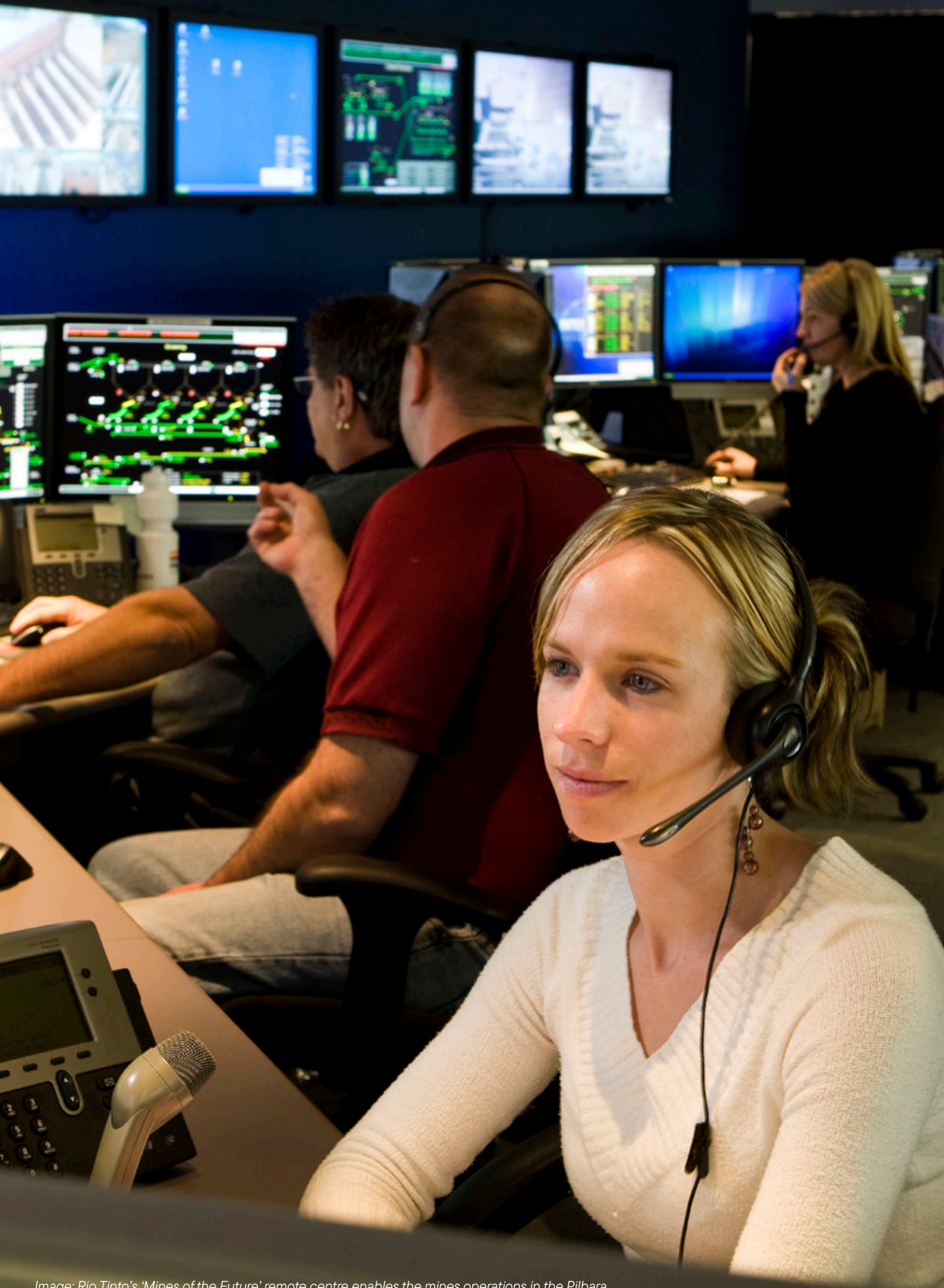
Image: Rio Tinto's 'Mines of the Future' remote centre enables the mines operations in the Pilbara to be controlled from one central location more than 1,000 kilometres away from the sites.
