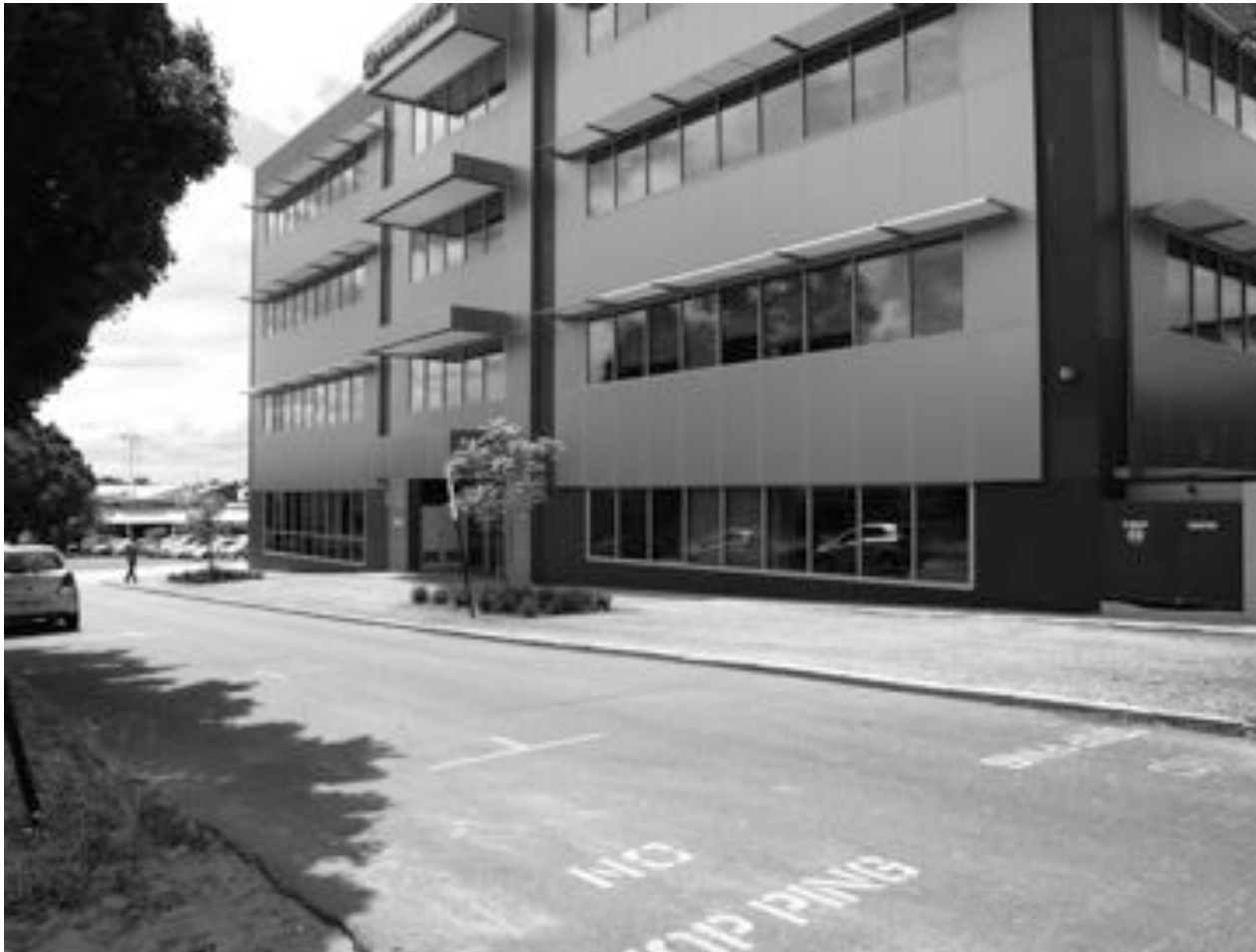
A new building meets the street, but still lacks pedestrian amenity. Note the shade structures over all the windows apart from the ground floor ones where the shade is needed most.
