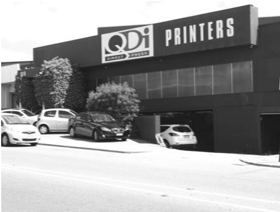
Car parking in the setback area is an unacceptable urban design outcome, regardless of whether it's done like this ...
