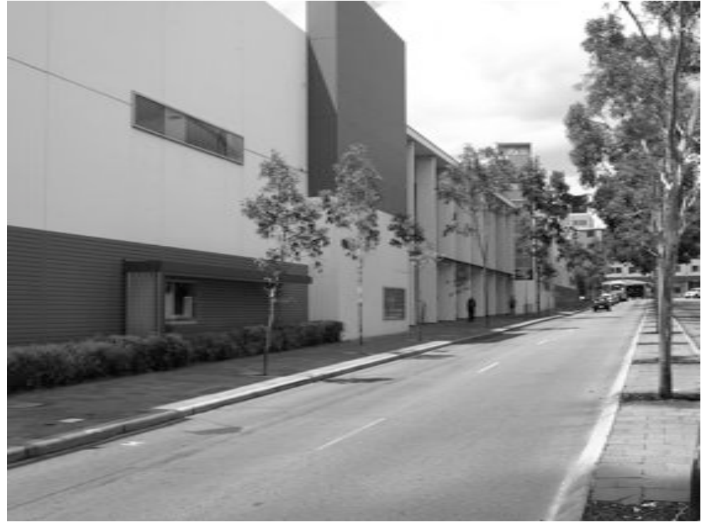
Retail as a land use does not guarantee good street. Note, this is an important pedestrian link back to the city centre.
