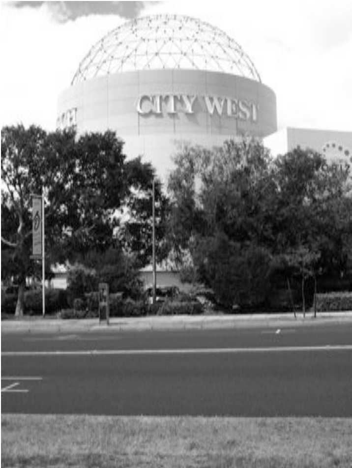
Whilst the dome is a landmark, it lacks architectural significance and is a landmark only by virtue of the fact that it isn't obscured by anything else.
