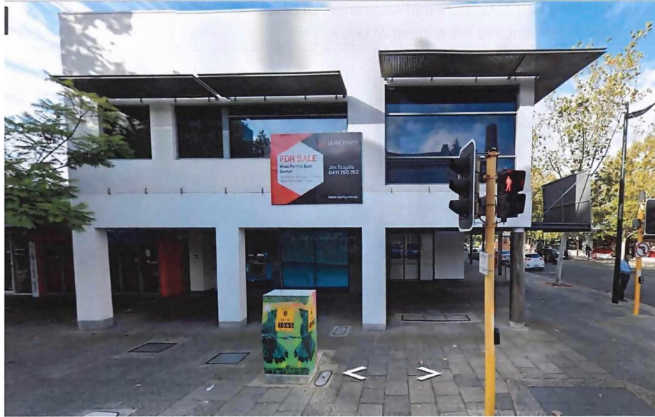
1275 Hay Street – Street View - Colonnade
