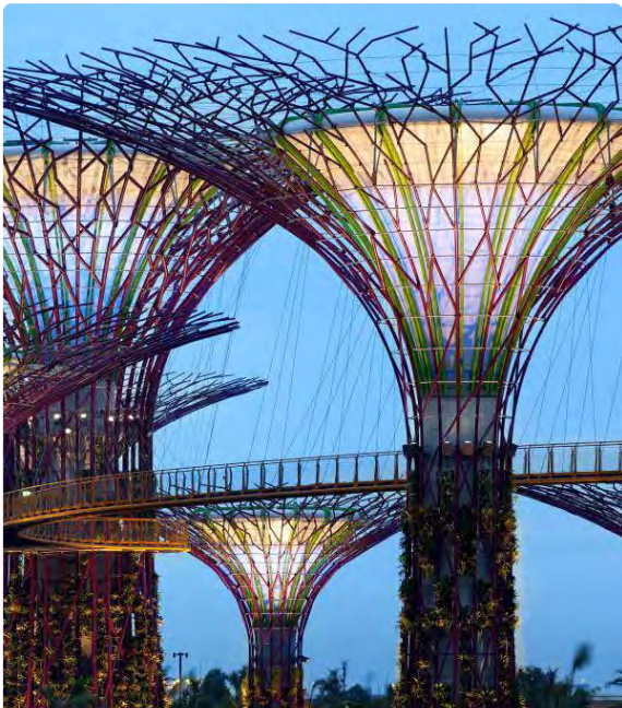
SCULPTURAL TREE WITH STEEL FRAME AND WIND ACTIVATED CHAIN MESH
