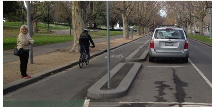
Example: granite kerb separator, Melbourne
