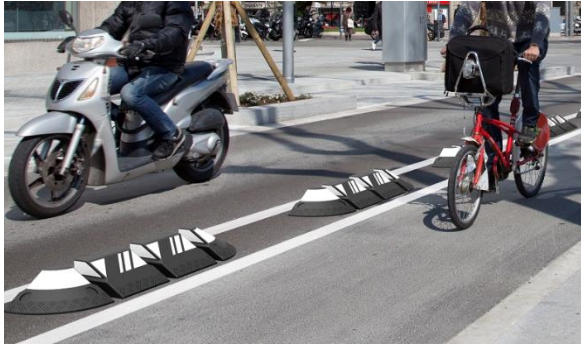
Example: Zipper kerb separator, Barcelona
