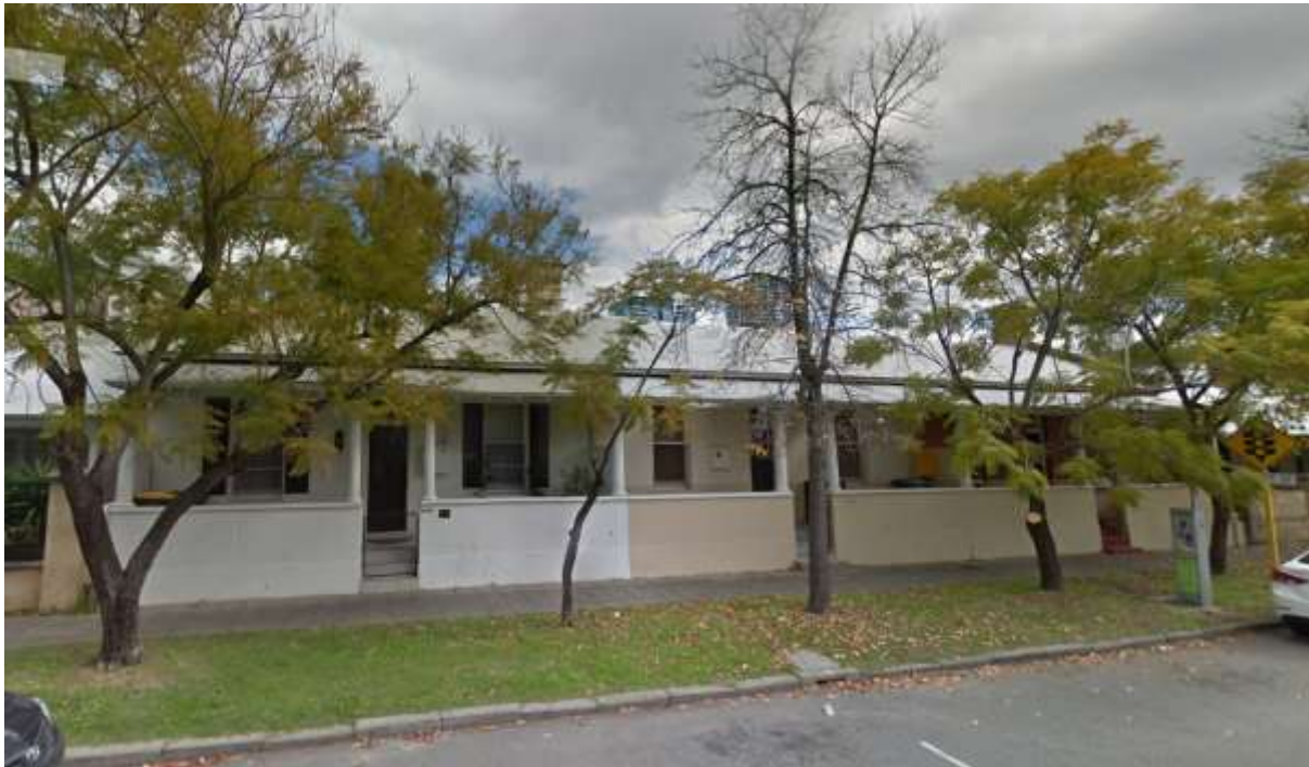
Existing verandah and façade
