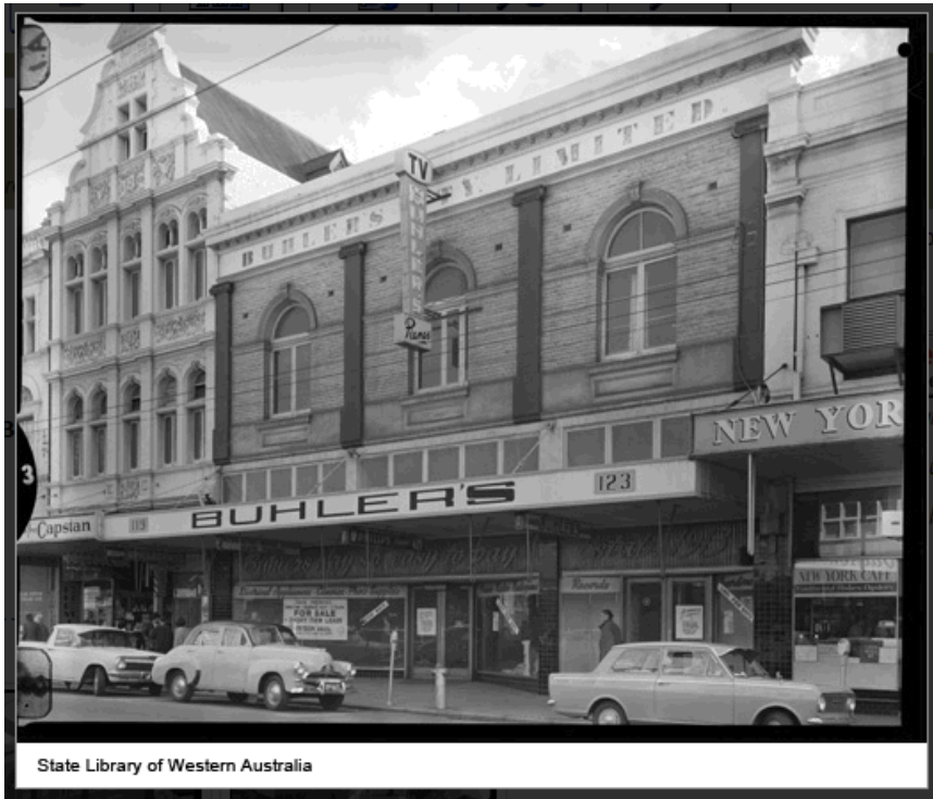
ORIGINAL TO BE REINSTATED
