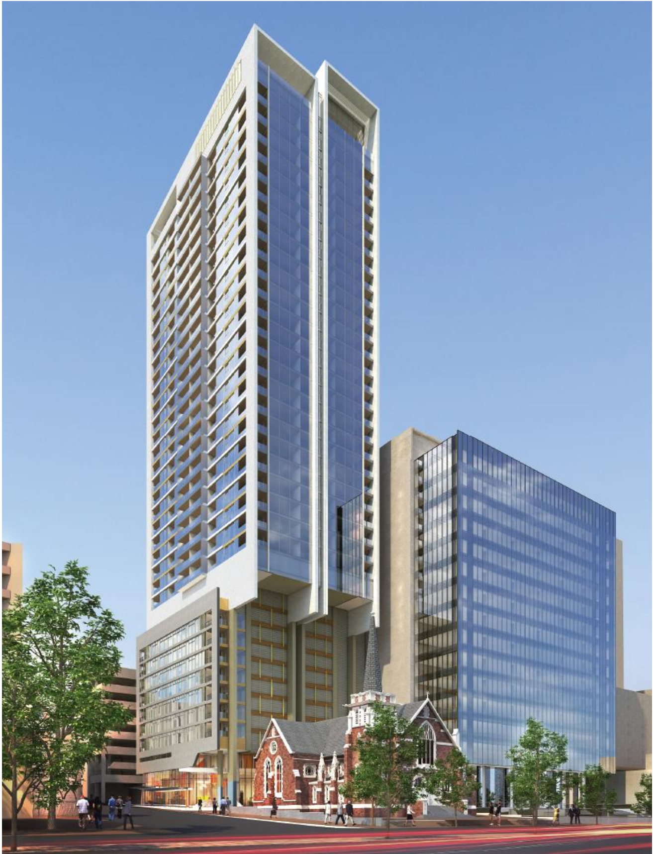
15/5201; 36 (LOT 18) ST GEORGES TERRACE & 10-14 (LOTS 19 & 50) PIER STREET, PERTH
